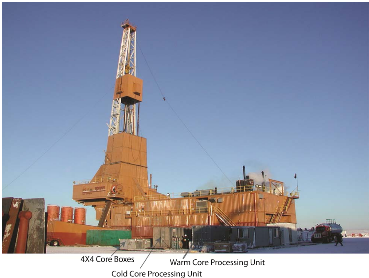
Figure 53: Doyon 14 rig and pipeshed during Mt Elbert-01 operations, Milne Point Unit, Alaska North Slope, February 2007
