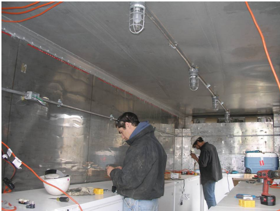
Figure 96: ASRC electrical and construction staff modifying core storage refrigerated unit for lighting, electrical outlet, and man-door. Extension cords visible in photo were for temporary power to freezers to keep core cold during unit modification (May 16, 2007).
