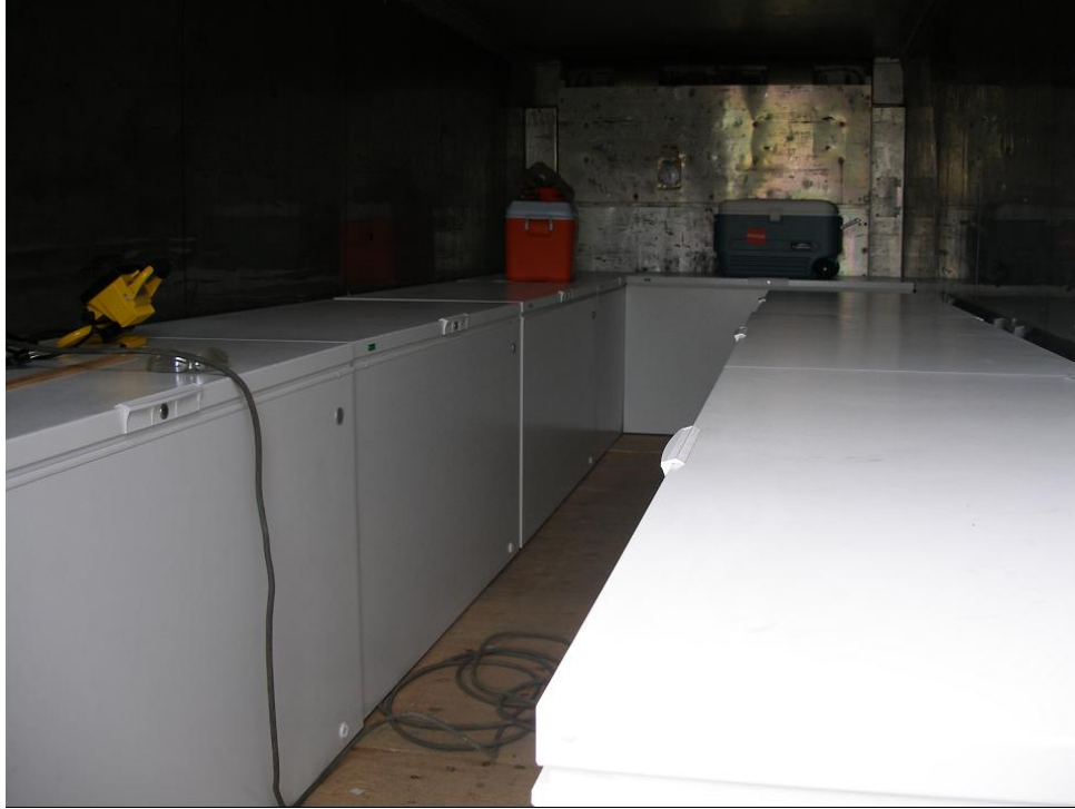
Figure 95: 6 of 8 Freezers installed for core storage in refrigerated unit prior to temporary disconnection of unit for installation of man-door, electrical outlets, and lighting (May 16, 2007)
